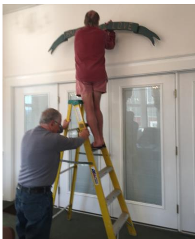
Painting is finished; time to restore the carving. Team work is essential! Thom and Gerry on hand to tackle what appears to be an easy job.
